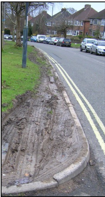
A damaged verge on Hillsway. A few people can spoil an area for everyone.
